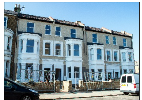
40-46 Sweyn Road, Cliftonville
