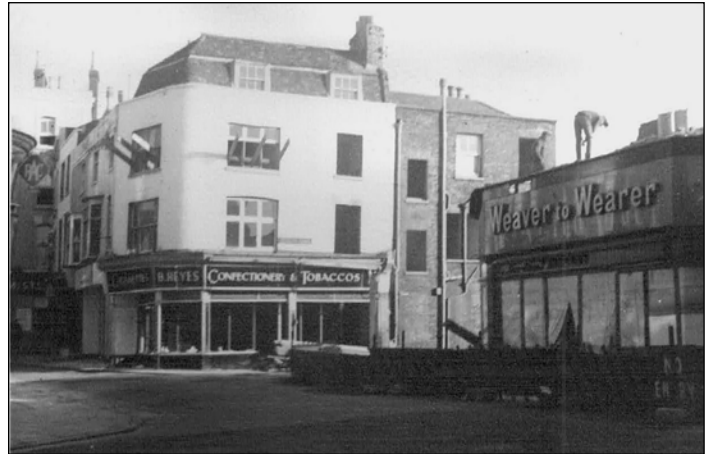
Shops at the junction of Queen Street and Wellclose Square before demolition - January 1968
