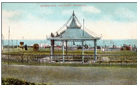
Bandstand, The Fort Showing lights being fitted
