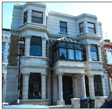
12 Arthur Road, Cliftonville
